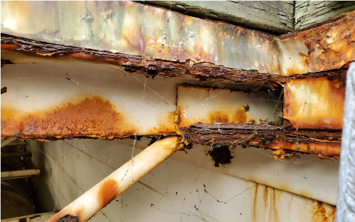
Figure 6 – Roof Joists at Access Hatch
