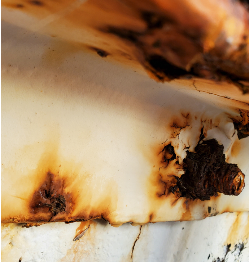
Figure 6 – Steel Angle Ledger at Wall
